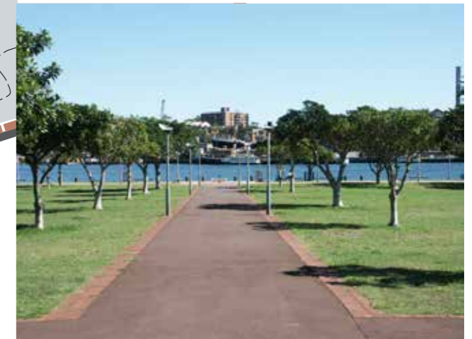
Red-brown bitumen as used at the Bi-centennial Park Glebe
