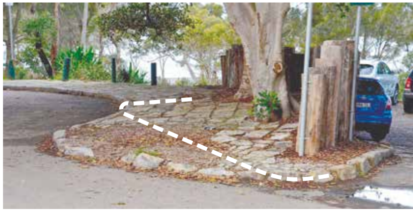
New sandstone kerb to roundabout-addressing truck movement patterns
