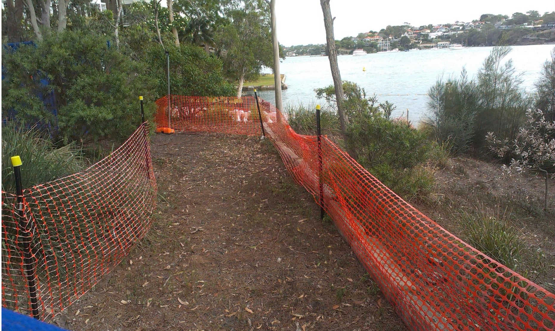
Middle level path toward foreshore, location for upper ramp of access ramp option
