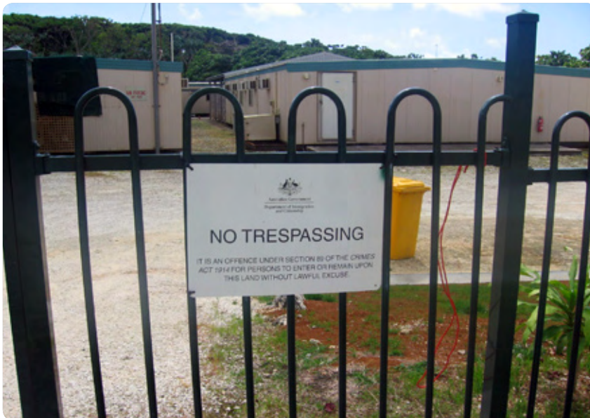
..... Construction camp immigration detention facility, external view
